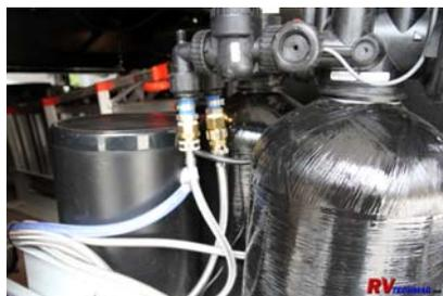
The stainless steel garden hoses were attached to the softener and clamped at the rear of the tray
