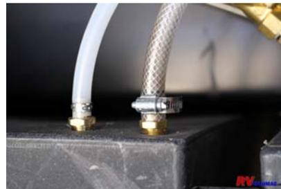
The polyvinyl drain hose for the softener was inserted into the top of the gray tank next to the braided clear vinyl drain line from the iron filter
