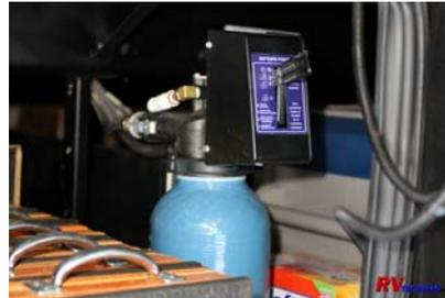
The iron filter was relocated to an available area to make room for the softener, brine tank and deionizer
